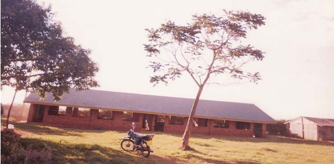
PHOTO 1: KIMLOT PRIMARY SCHOOL
