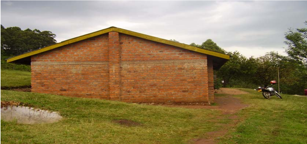
PHOTO 1: KOMOTOBU SECONDARY SCHOOL
