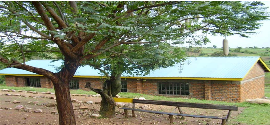
PHOTO 2: KOMOTOBU SECONDARY SCHOOL
