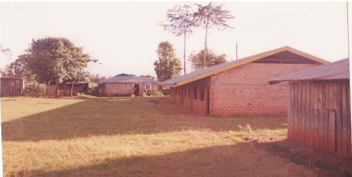
PHOTO 2: KIMLOT PRIMARY SCHOOL
